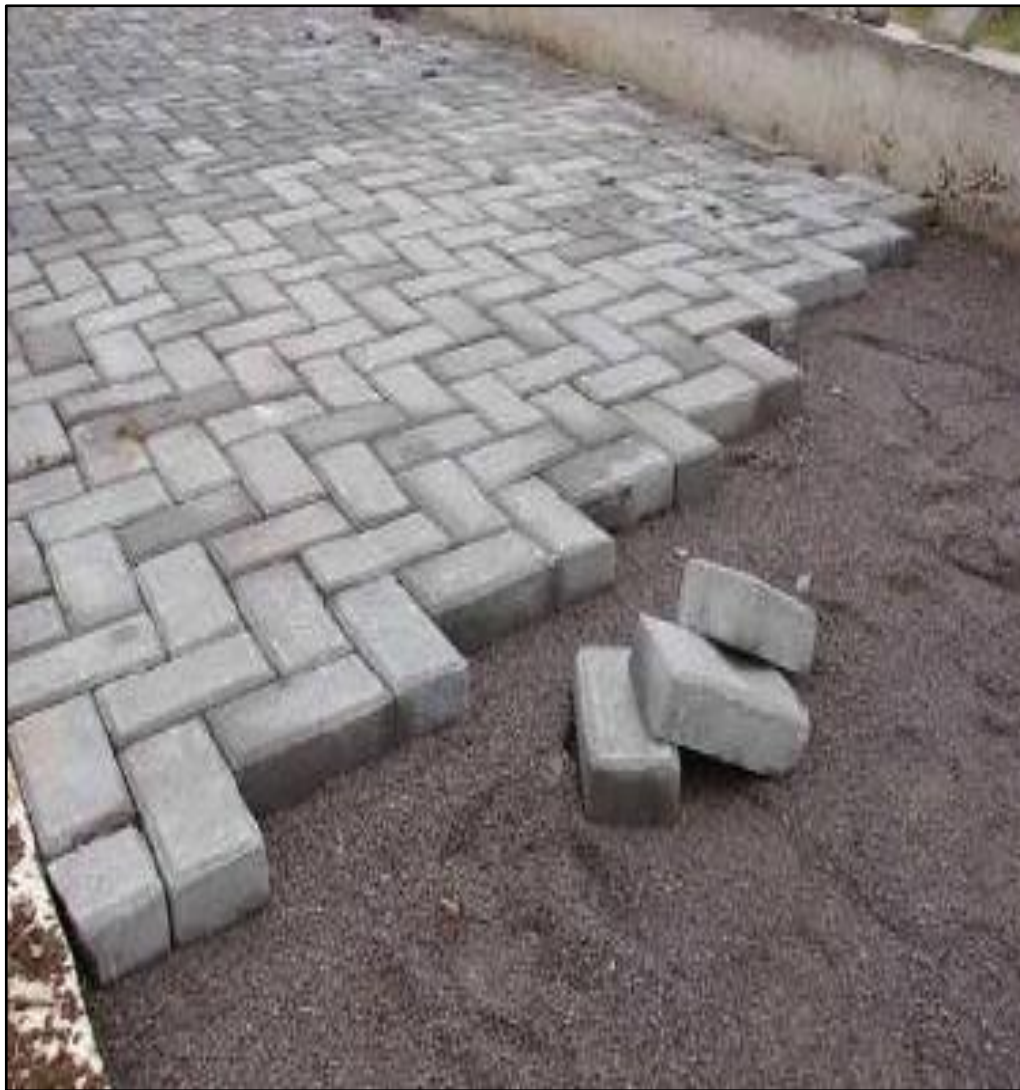
Figure 10. Concrete blocks interlocked sitting on sand cradle Source: Virgiliis, 2009.
