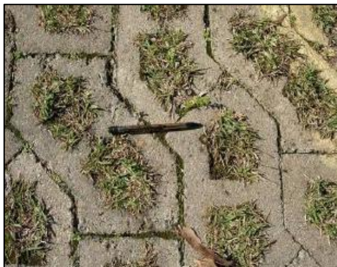
Figure 9. Concrete blocks precast hollow. Virgiliis 2009 Source
